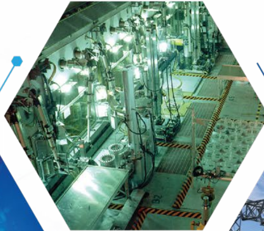
Materials and Fuels Complex
